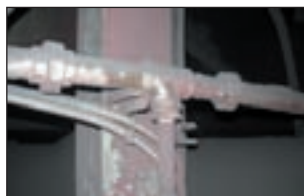
Old valves system
