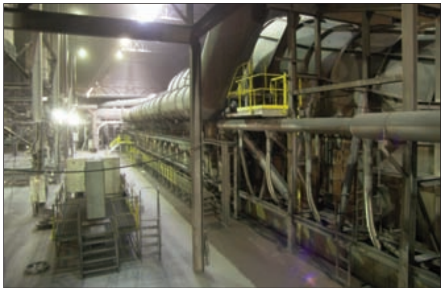
Indurating Machine #3 - South Side Burner Floor.
