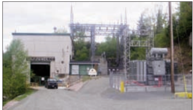
SM2's new outgoing transformer.
