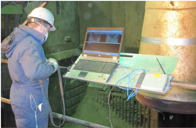
Ron Fitzgerald ; Maintainer Operator Mechanical 2, conducting the installation of the mantle using the new camera system
