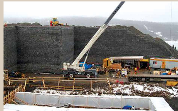
The wall surrounding the new crusher
