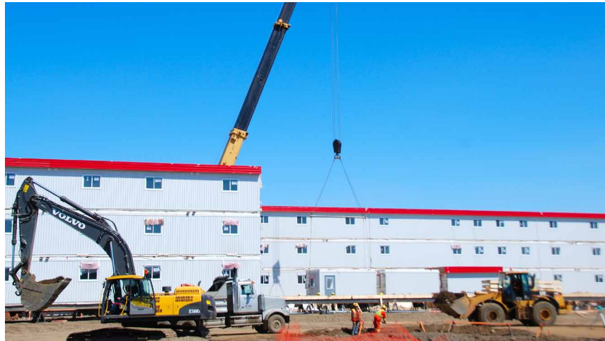
Sustaining Capital Dorms – Labrador City Industrial Park
