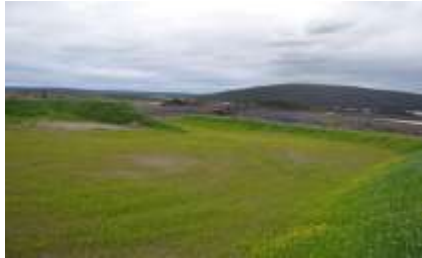
Beaver Bay Stock Pile rehabilitation
